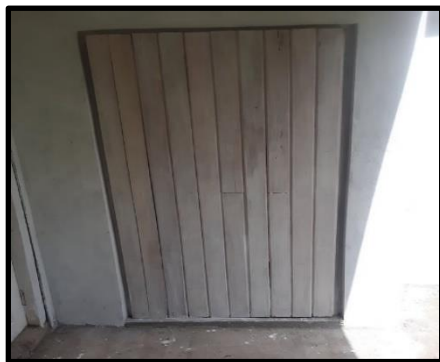
Storage room completed, except for painting.
