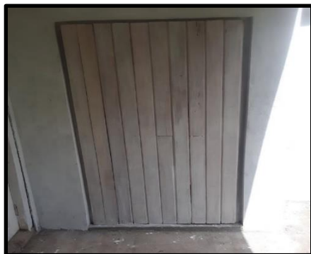
Storage room completed, except for painting.
