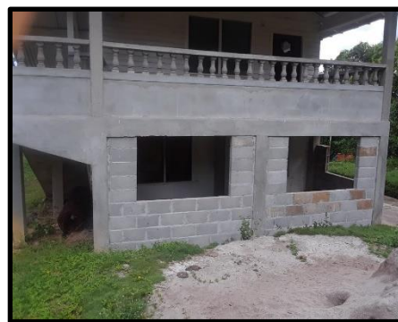
An incomplete extension of the Bible School Room.
